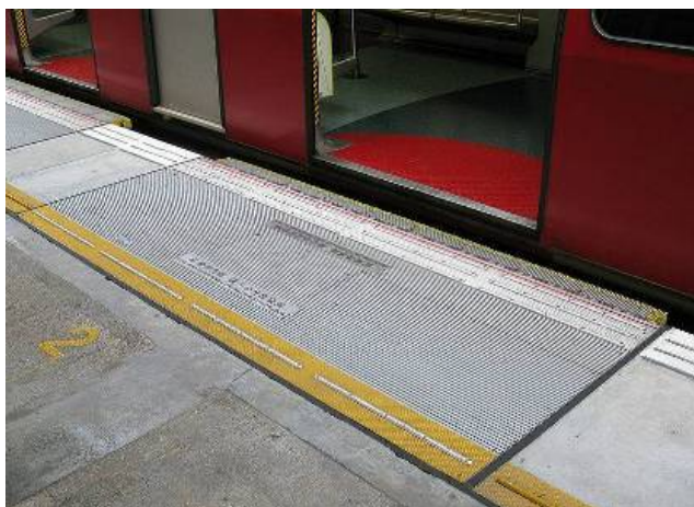
Figure 21: Platform gap filler in Hong Kong
