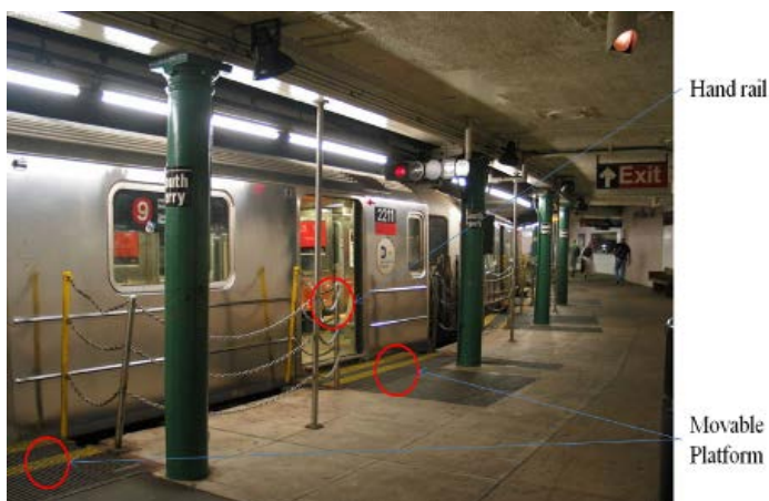
Figure 22: Platform edge extender at South Ferry, USA
